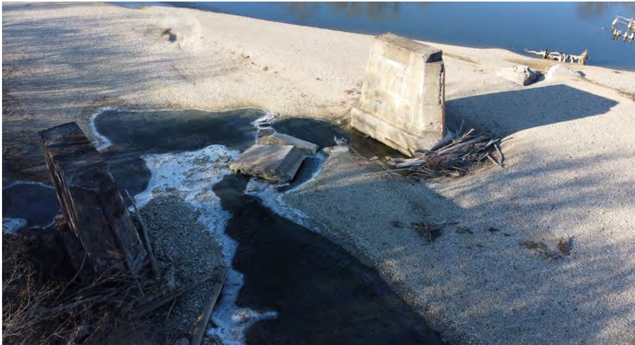
Bridge 184 piers from a drone perspective - photo provided by Jim Krause
