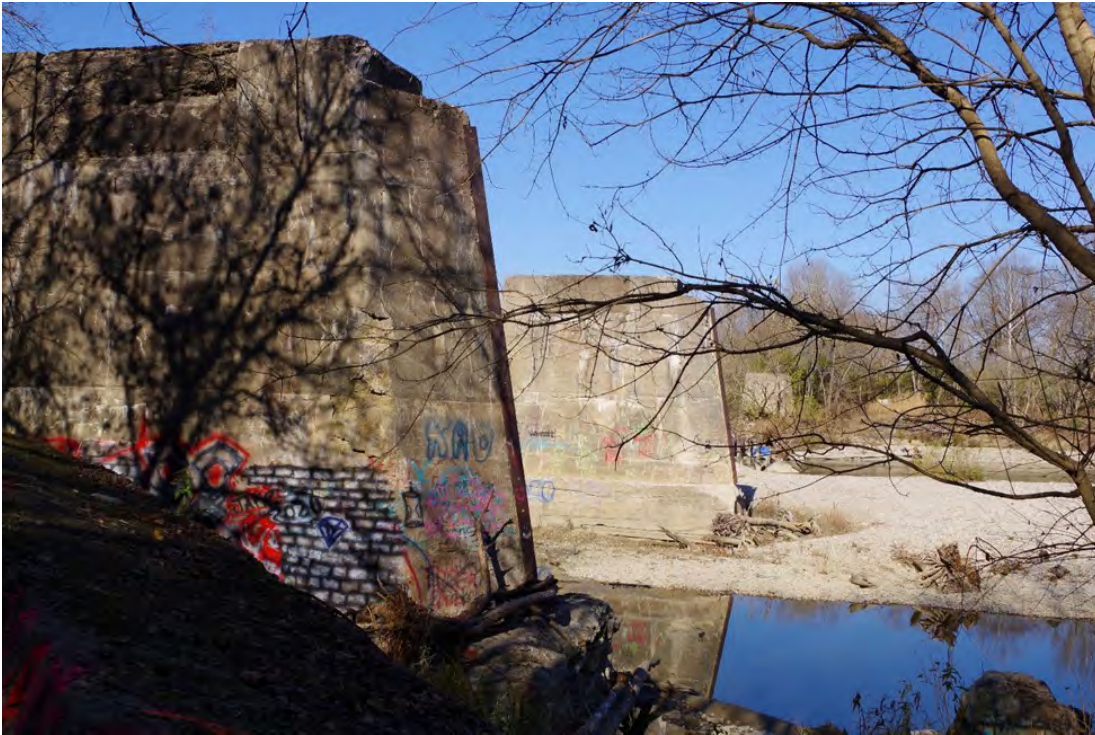
Remaining Bridge 184 piers in current state — photo provided by Jim Krause
